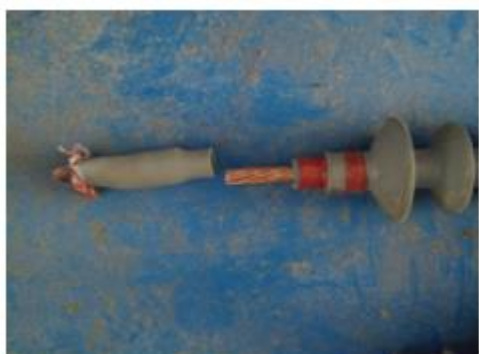
Fig. 8 Cable Pulling physical map
