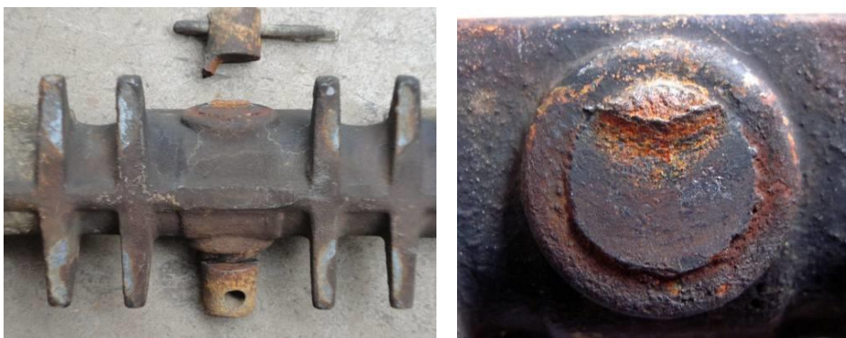
Fig 2 Fracture # 42 suspension clamp Fig 3 # 42 bar suspension clamp fracture
