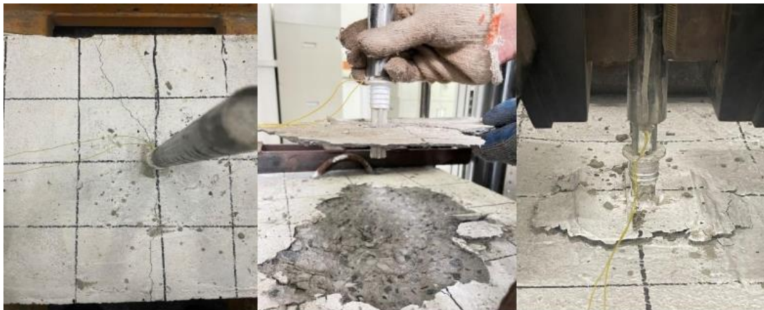
Fig. 7 ST1 ~ 3 Damage Phenomenon
