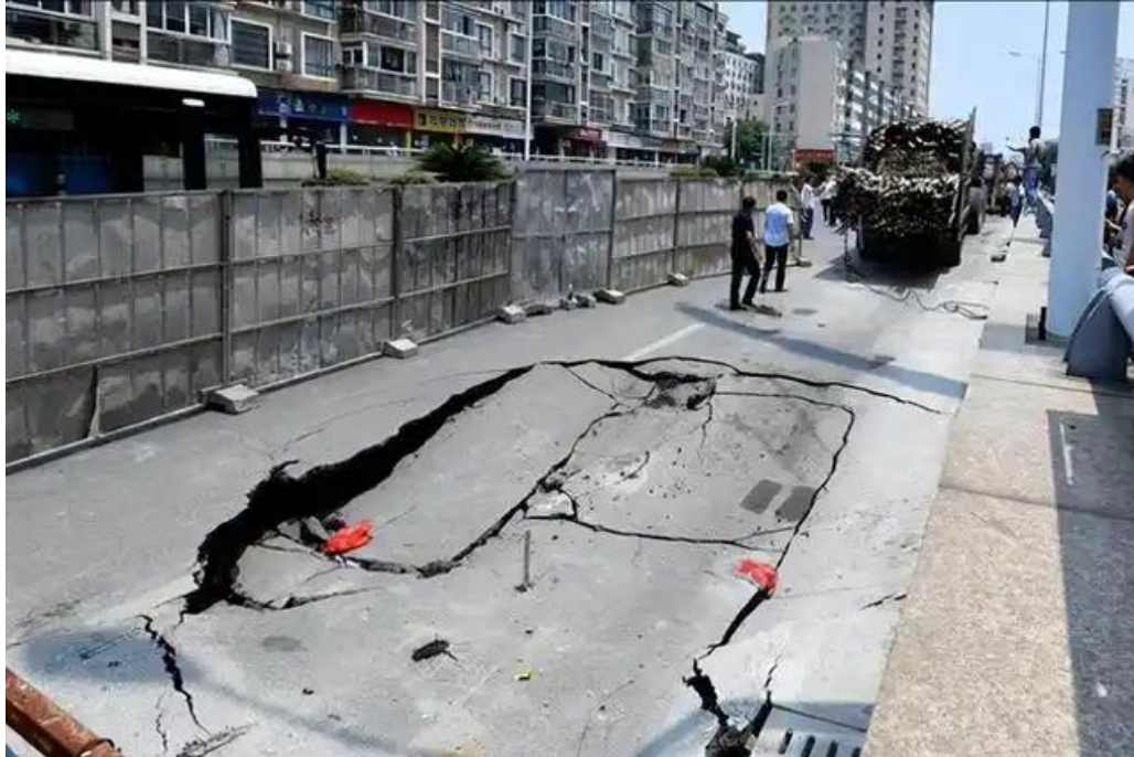
Fig. 5 Ground settlement and building damage
