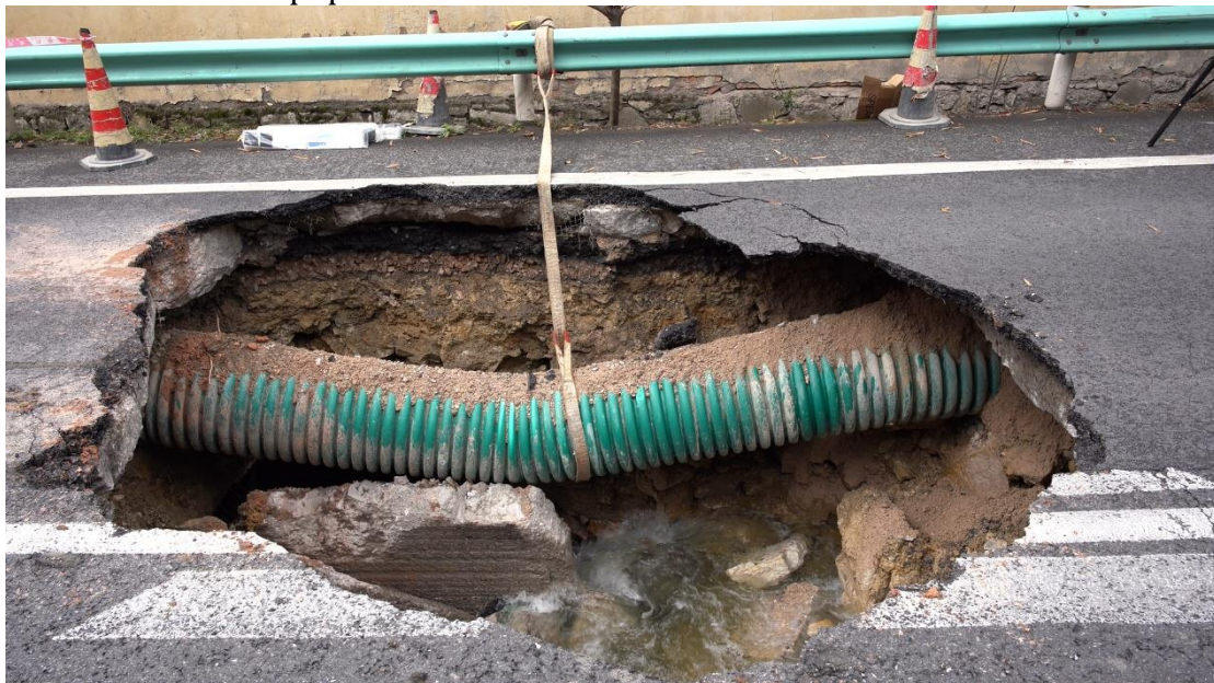
Fig. 2 Ground Subsidence Mechanisms Induced by Existing HDD Boreholes
