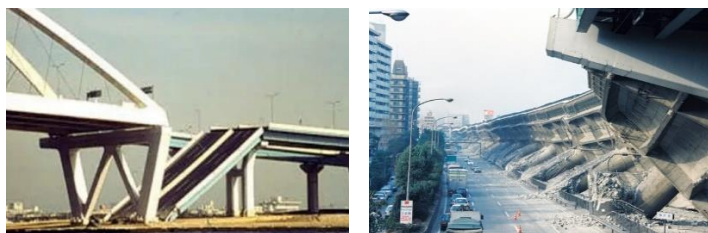
Figure 1: Beam damage caused by the Hanshin earthquake
