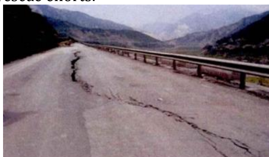
Figure 2: Damage to roadbeds caused by the Wenchuan earthquake
