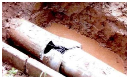
Figure 3 Damage to water supply pipes during an earthquake
