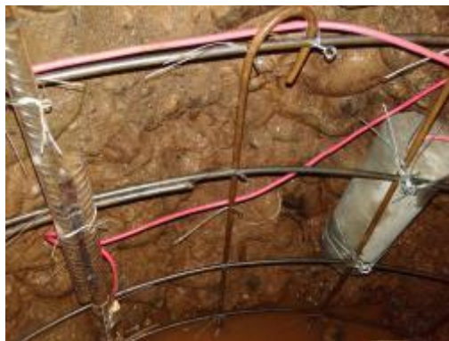
Fig.5 On-site installation of monitoring equipment
