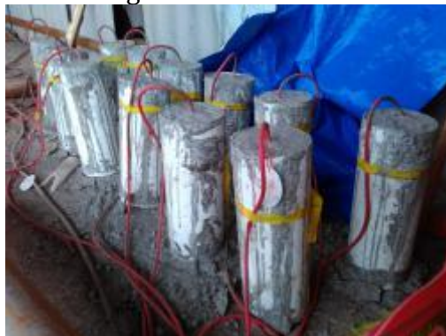
Fig.4 Protection before concrete meter installation
