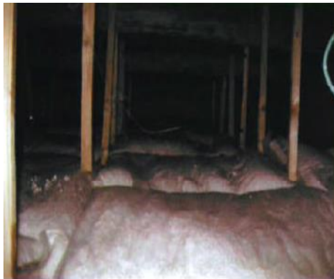
Figure 2: The ceiling laid insulation package
