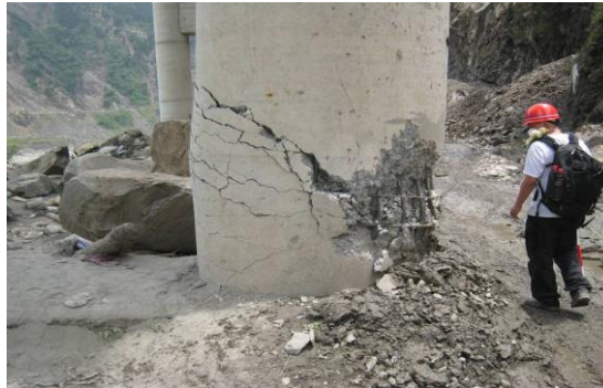
Fig 1. The damage of lowering of girder
