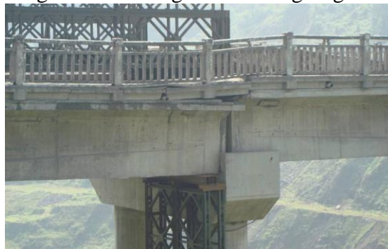
Fig 2. The damage of bridge pier
