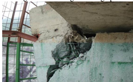
Fig 3. The damage of bridge abutment
