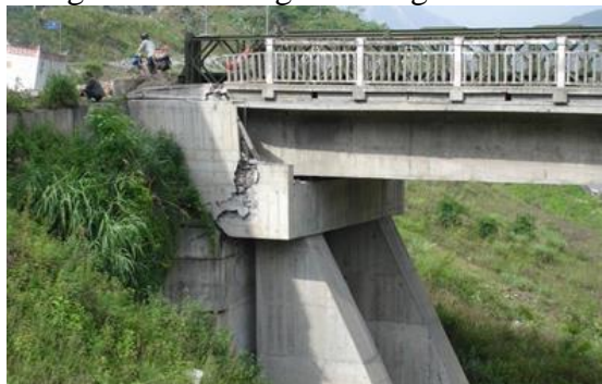
Fig 4. The damage of rubber plinth
