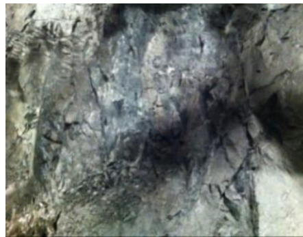
Figure 8: Tunnel face at ZK52+754
