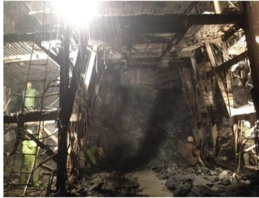
Figure 12: Water outburst at ZK53+021 crown left side
