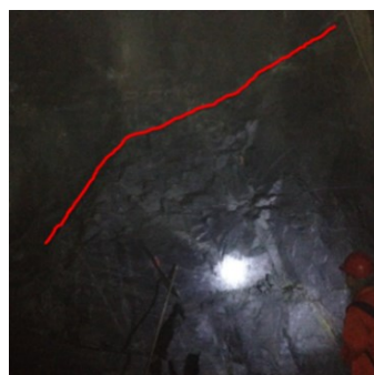
Figure 4: Tunnel face at ZK53+037
