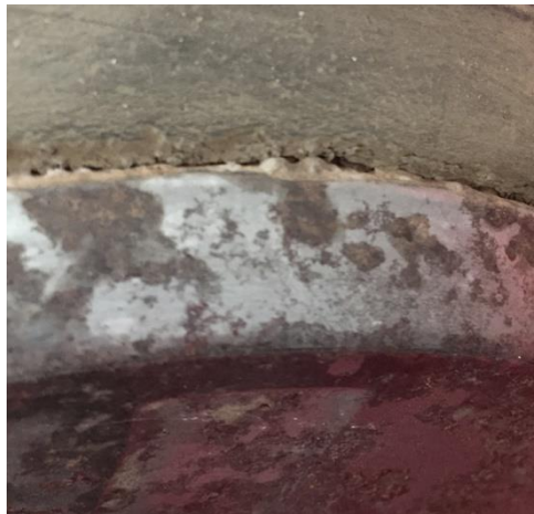
Fig. 2 The drilling pump valve body sealing hole fall off
