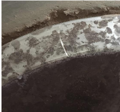
Fig. 1 The drilling pump valve body sealing block off
