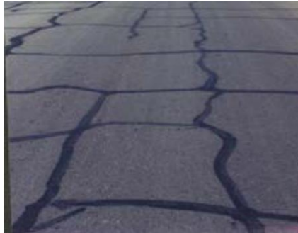
Fig.1 Block Cracking in HMA with Stabilized Base (Scullion 2002)
