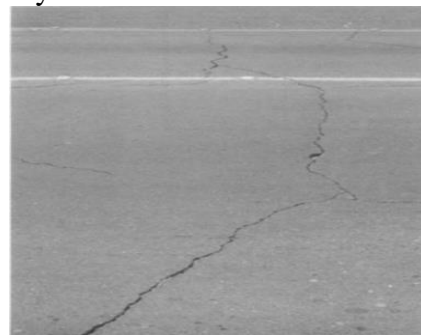
Fig.2 Transverse Cracking due to Shrinkage Cracking of CSL (Freeman and Little2002)
