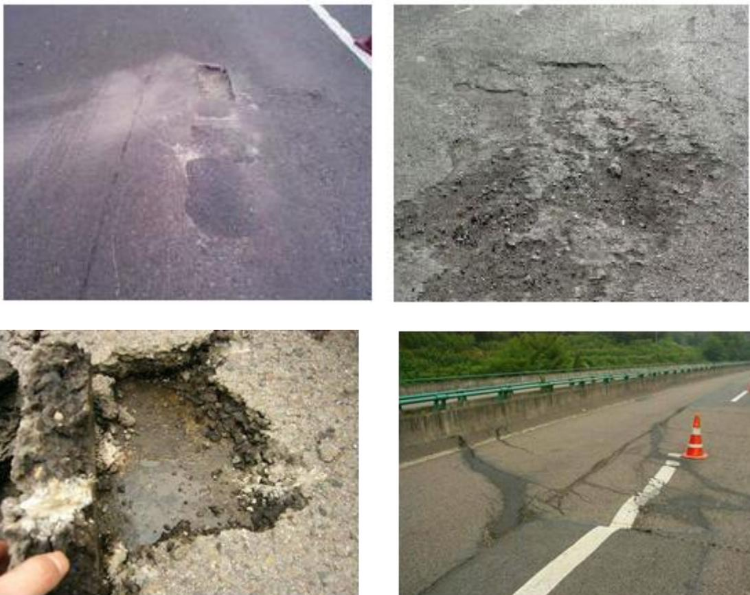
Fig.1 Water damage representative form of pit slot
