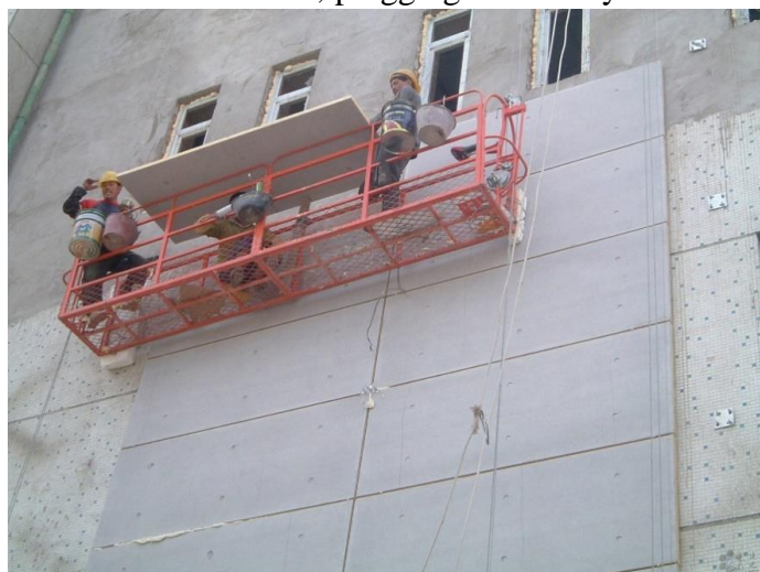
Figure 3 insulation construction of high-rise building
