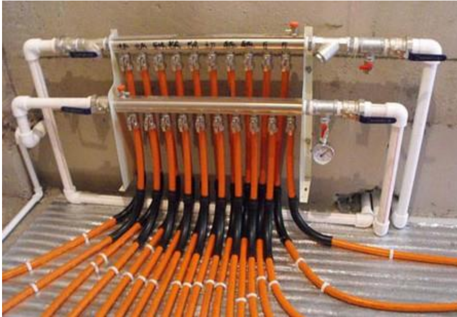
Figure 1 -rise building HVAC piping installation
