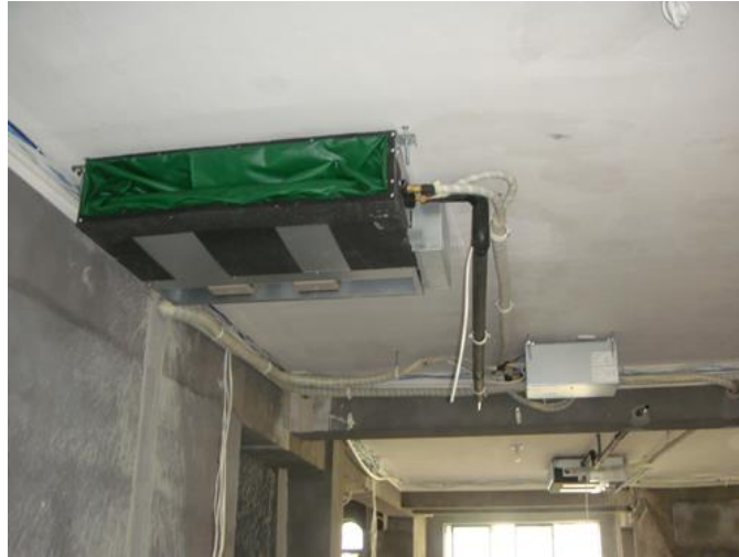
Figure 2 central air conditioning air outlet installation
