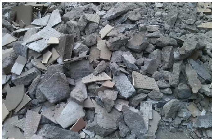
Fig.1 The construction waste formed at the time of building demolition
