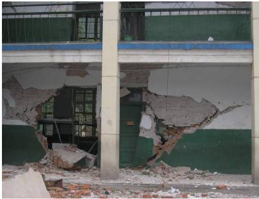
Figure 1 Longitudinal wall failure Figure 2 Oblique cracks in the wall of the door
