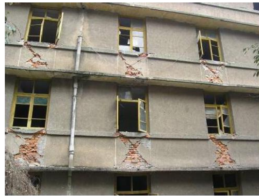
Figure 3 X - shaped cracks in the wall between windows and under the window
