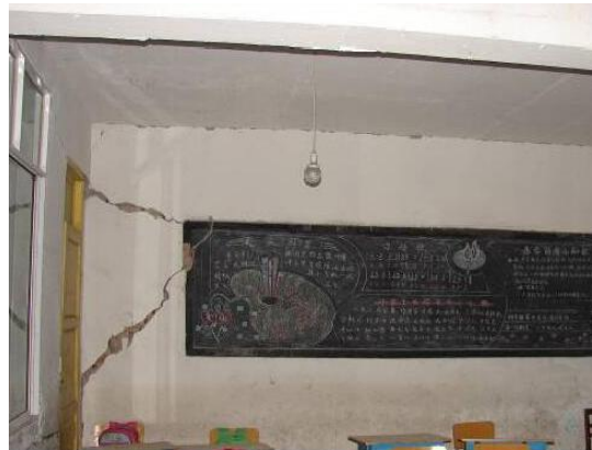
Figure 4 diagonal cracks in the cross wall
