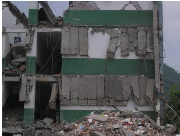
Figure 7 The collapse of the wall causes the precast slab to fall off
