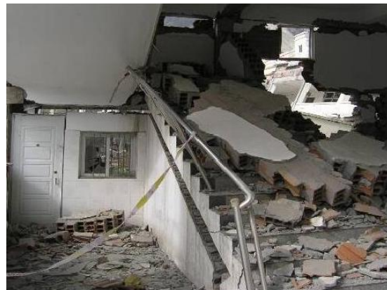
Figure 6 Collapse of stairs
