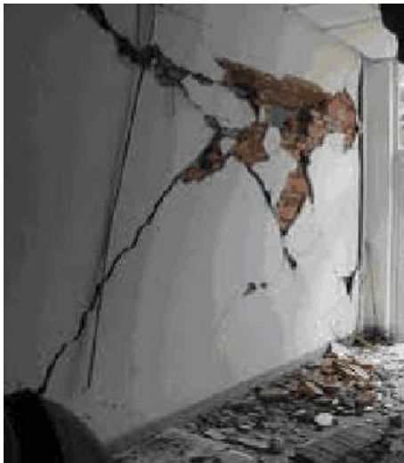
Figure 5 x- shaped cracks in the cross wall
