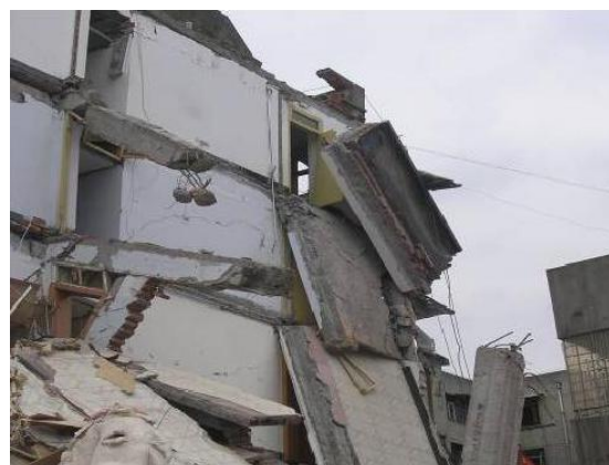
Figure 9 The collapse of parapet wall
