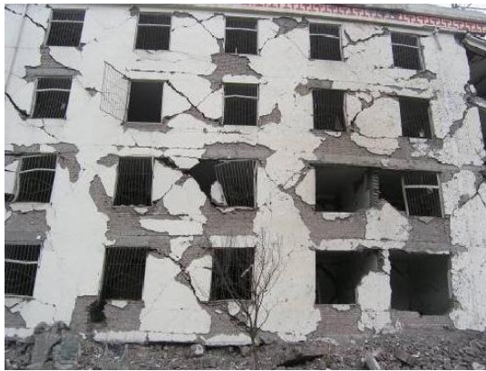
Figure 3 X - shaped cracks in the wall between windows and under the window
