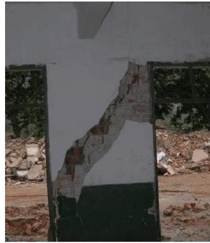
Figure 1 Longitudinal wall failure Figure 2 Oblique cracks in the wall of the door
