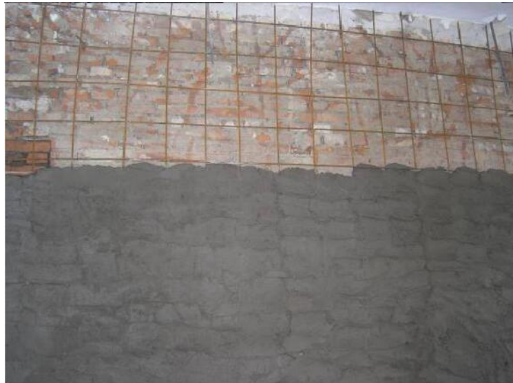
Figure 11 The field practice of coating cement mortar with steel meshes
