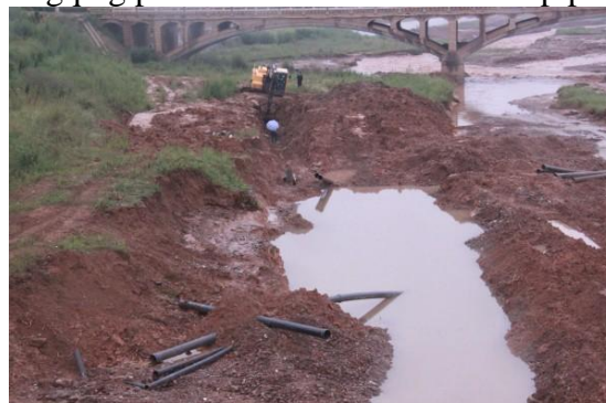
Fig.2 A damaged site
