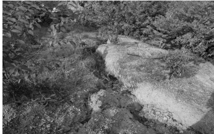
Fig.3 Slope damage of the flood
