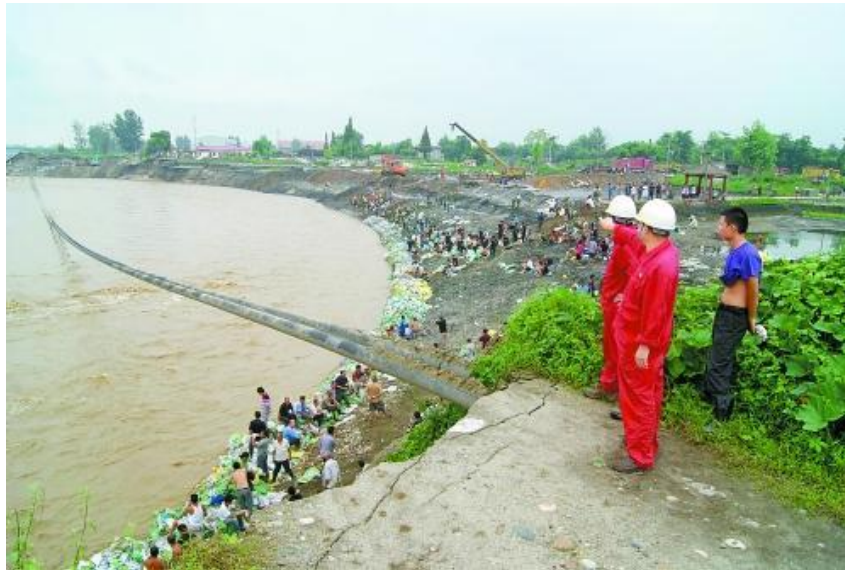
Fig.5 ditches damage of flood
