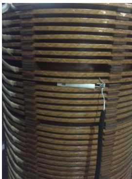
Fig. 7 Placement of the PD source outside the high voltage winding
