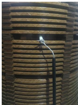
Fig. 9 Placement of the PD source inside the high voltage winding
