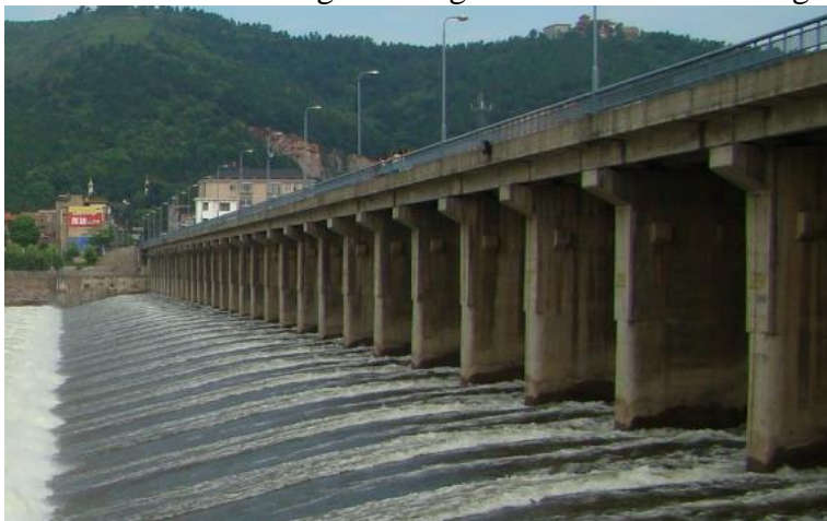
Figure 3 North Gate of the 54 hole of apron
