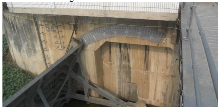
Figure 2 Flood diversion sluice
