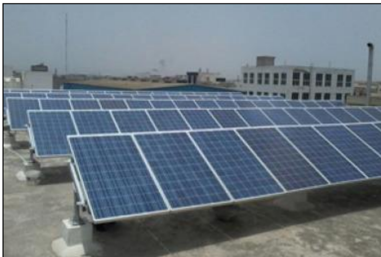
Figure 2- 6| Rooftop Solar Project.
