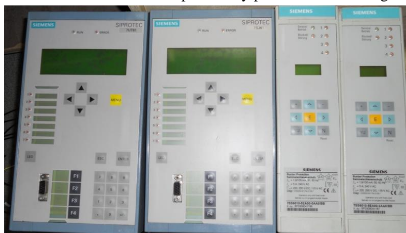
Fig 4. A microcomputer relay protection device
