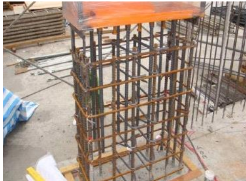
Fig.1 Reinforcement lap connection
