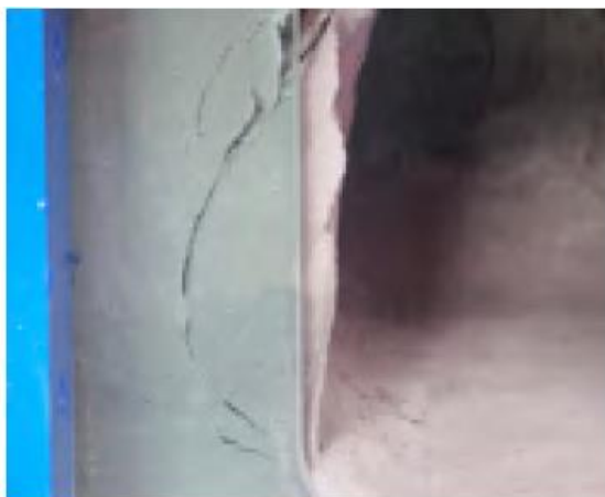
Wide shear crack formed on left sidewall of 40cm cavern
