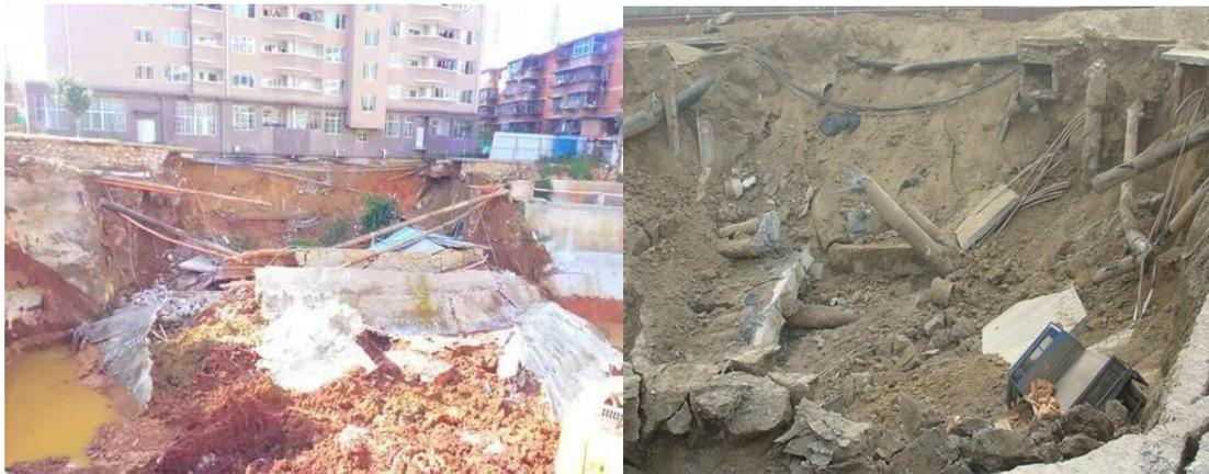
Fig.1 The collapse map of the foundation pit at the construction site
