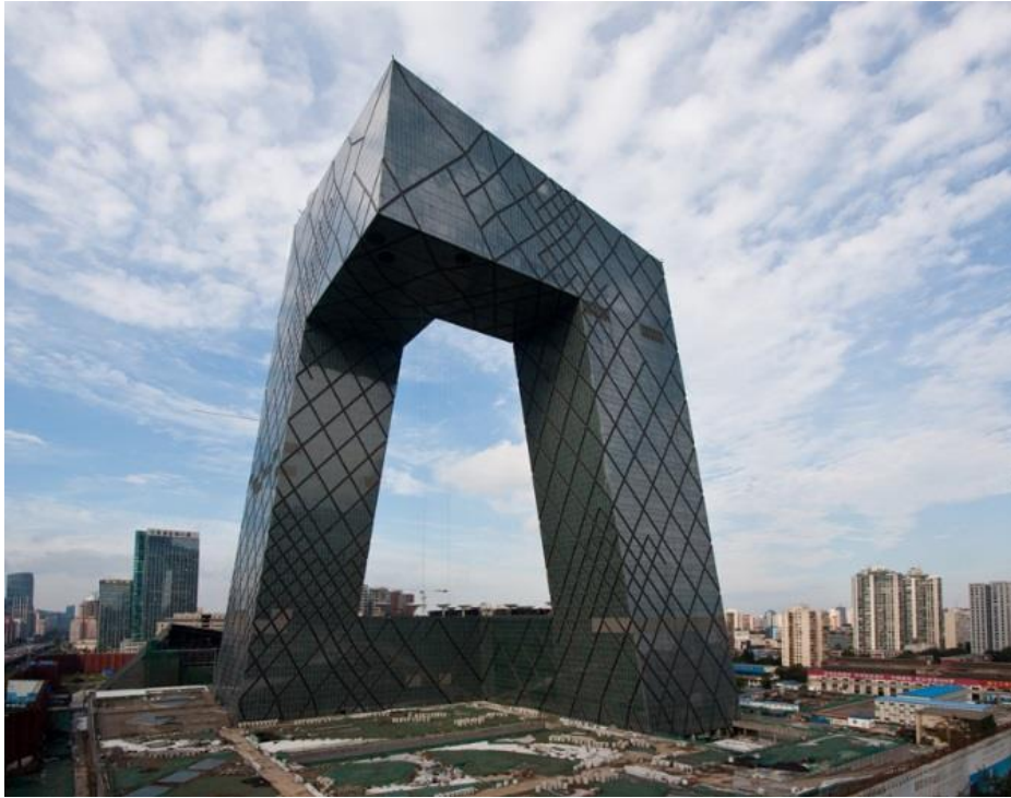
Fig. 1 The CCTV Headquarters
