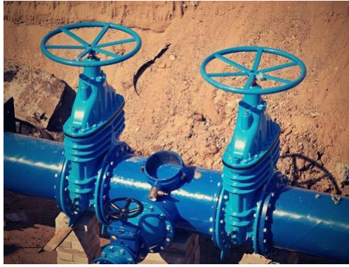
Figure 3: Natural gas pipeline valve
