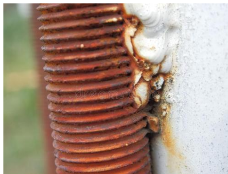
Figure 4: Pipeline thread corrosion
