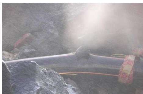
Figure 1: Leakage of natural gas pipeline
