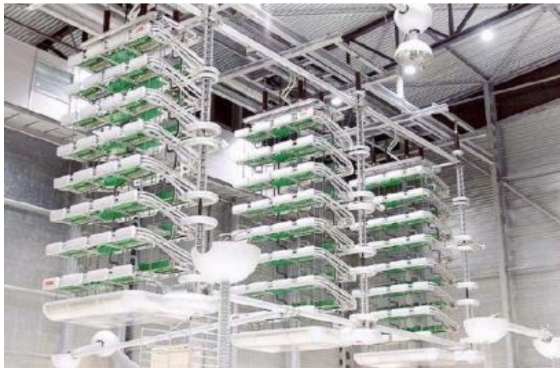
Fig. 1 Thyristor valve
