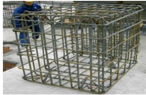
Fig. 2 Reinforcement of pile cap
